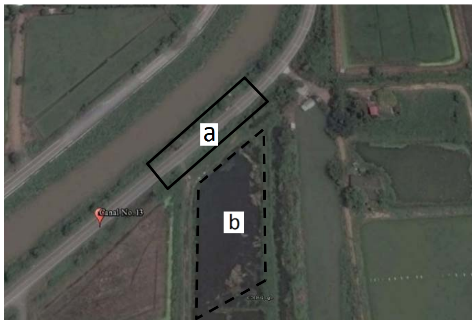
Fig. 2 a. The collapsed areas b. Shrimp ponds
