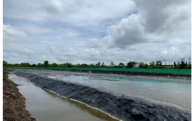
Figure 9. Site during operation of pumps
