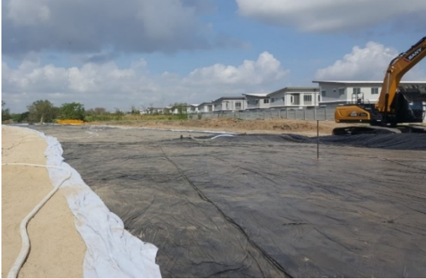
Figure 8. Spreading of geotextiles and sealing trench excavation
