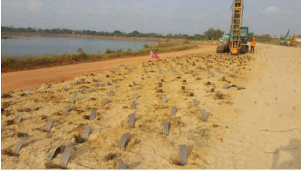
Figure 6. Installation of PVD using installation rig
