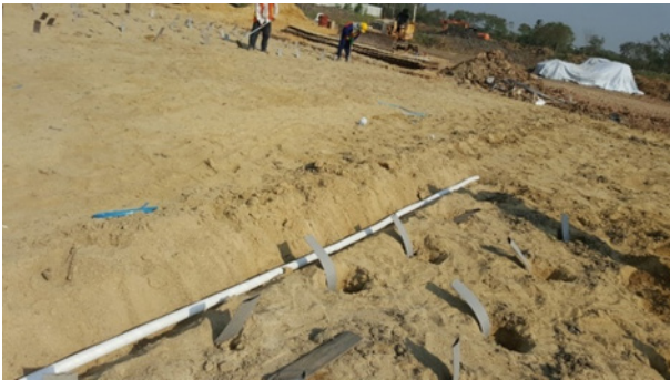
Figure 7. Installation of perforated horizontal drains
