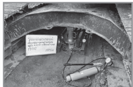
Plate Bearing Test
