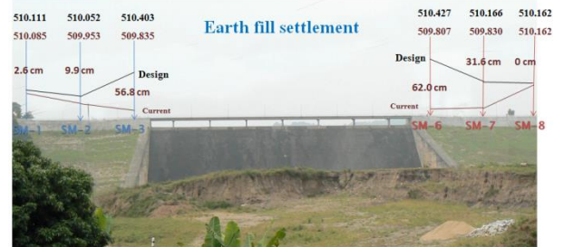
Figure 5 The settlement of the RCC section and earth fill
