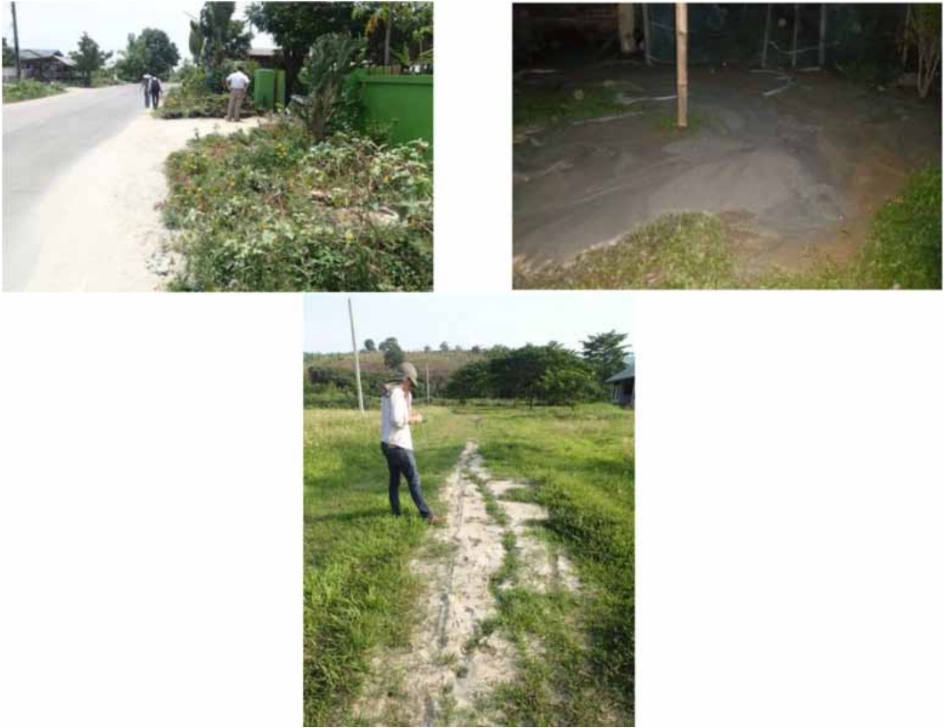
Figure 1. (a) Liquefaction at the edge of the road, (b) liquefaction-induced soil boiling (c) liquefaction on the paddy field
