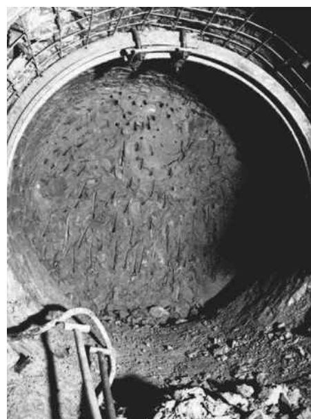
Figure 3. Circular adit used in backanalyses of the earth pressure coefficient at rest K_0 (Pavlik et al., 2004).
