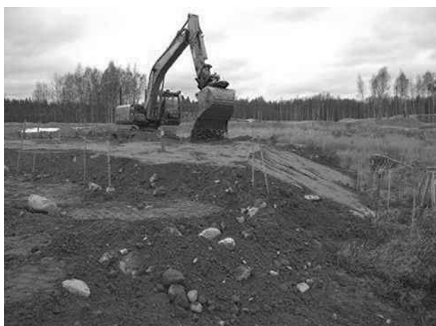
Figure 5 Construction up to height 1.5 m for embankment 1.
